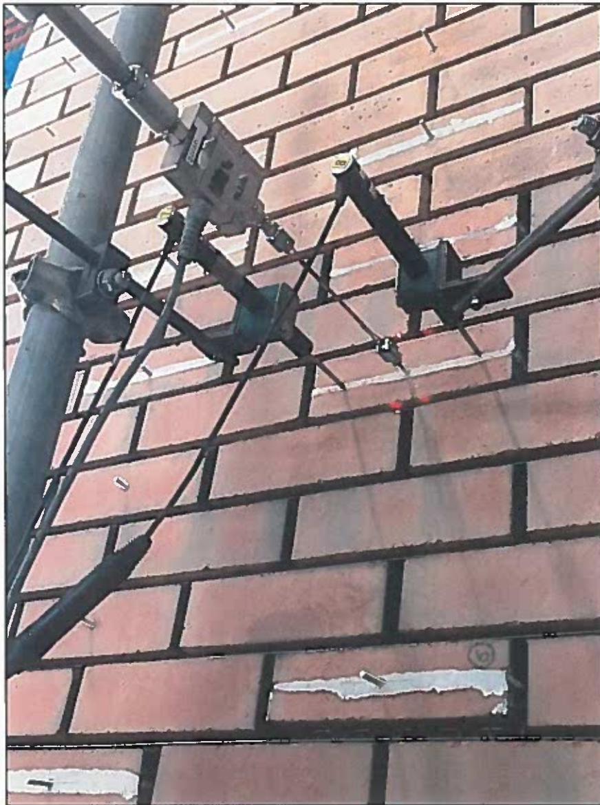
EXAMPLE OF PULL-OUT TEST SETUP
