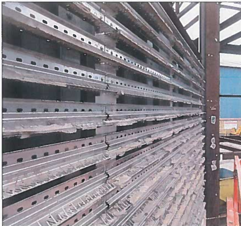
TEST SAMPLE DURING DISMANTLE
