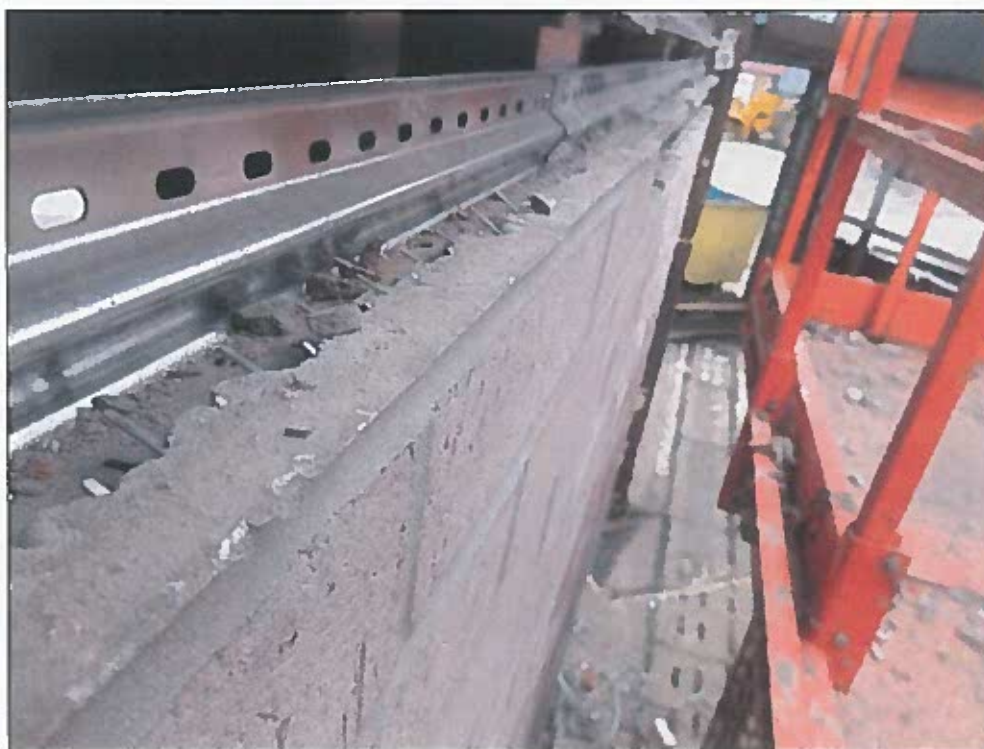
TEST SAMPLE DURING DISMANTLE
