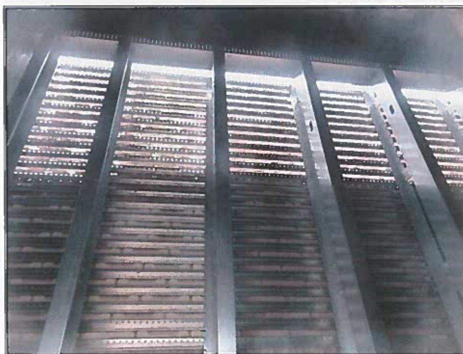
TEST SAMPLE DURING DISMANTLE
