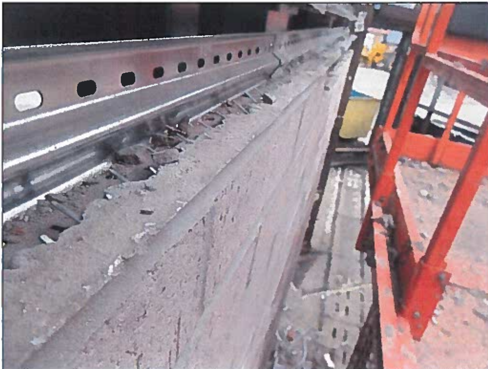
TEST SAMPLE DURING DISMANTLE
