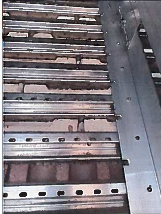
INTERNAL VIEW DURING WATER TEST
