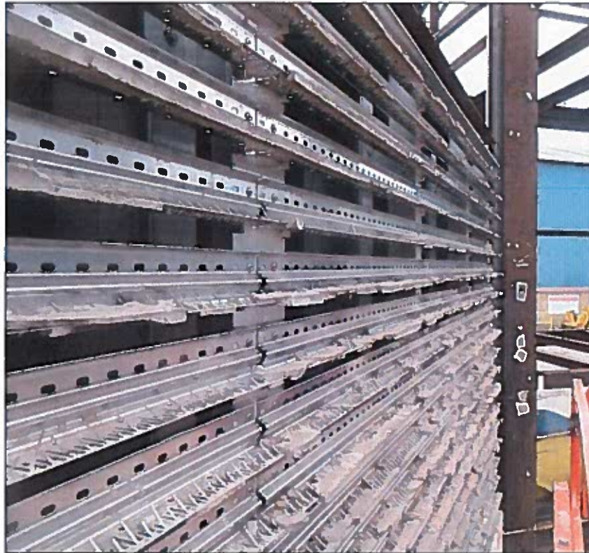
TEST SAMPLE DURING DISMANTLE
