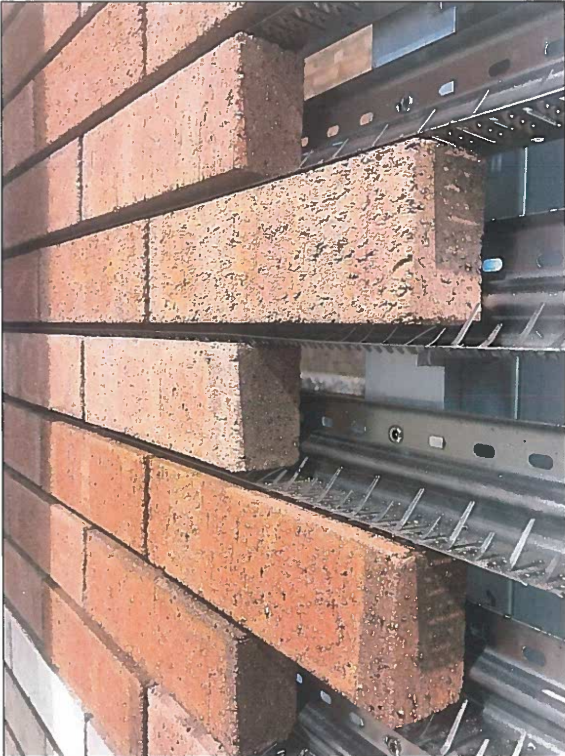
CLOSE UP OF BRICK SLIPS
