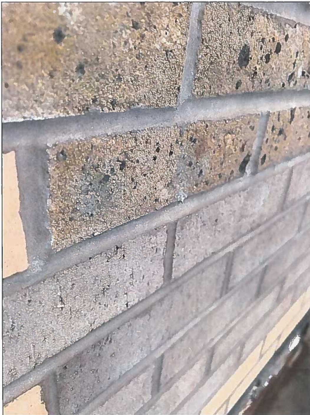
CLOSE UP OF BRICK SLIPS
