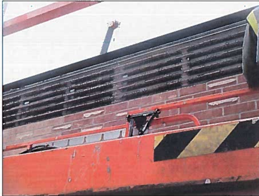
TEST SAMPLE DURING DISMANTLE
