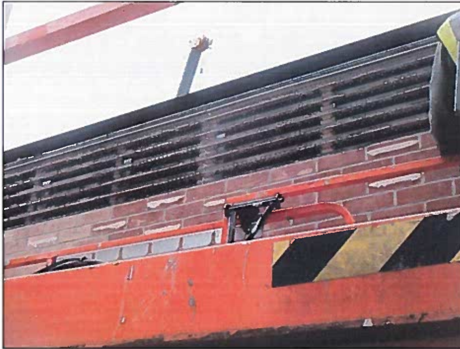
TEST SAMPLE DURING DISMANTLE
