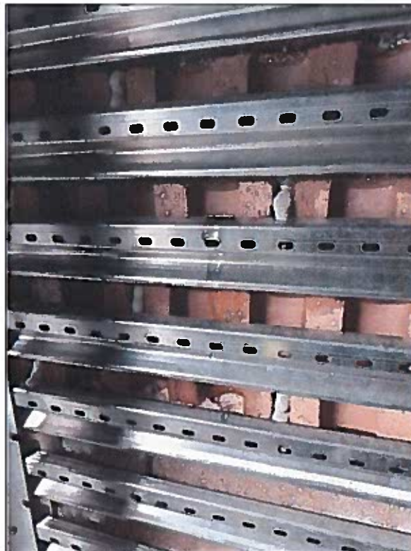
INTERNAL VIEW DURING WATER TEST
