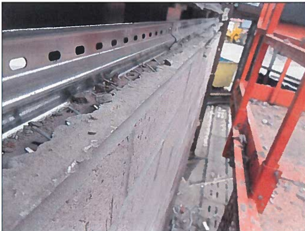
TEST SAMPLE DURING DISMANTLE
