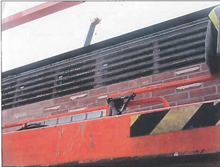
TEST SAMPLE DURING DISMANTLE
