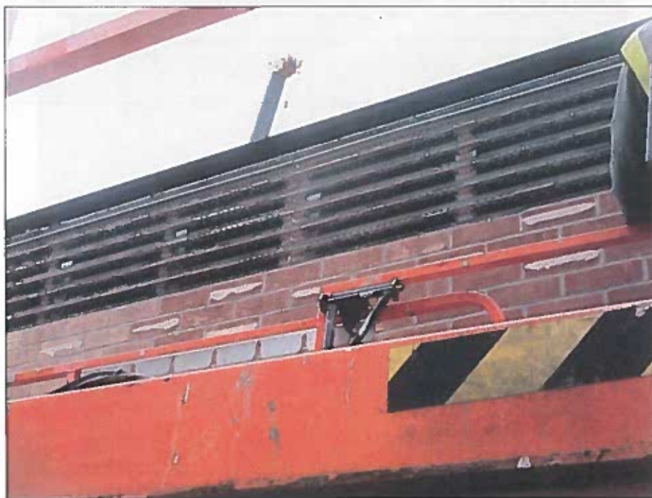
TEST SAMPLE DURING DISMANTLE
