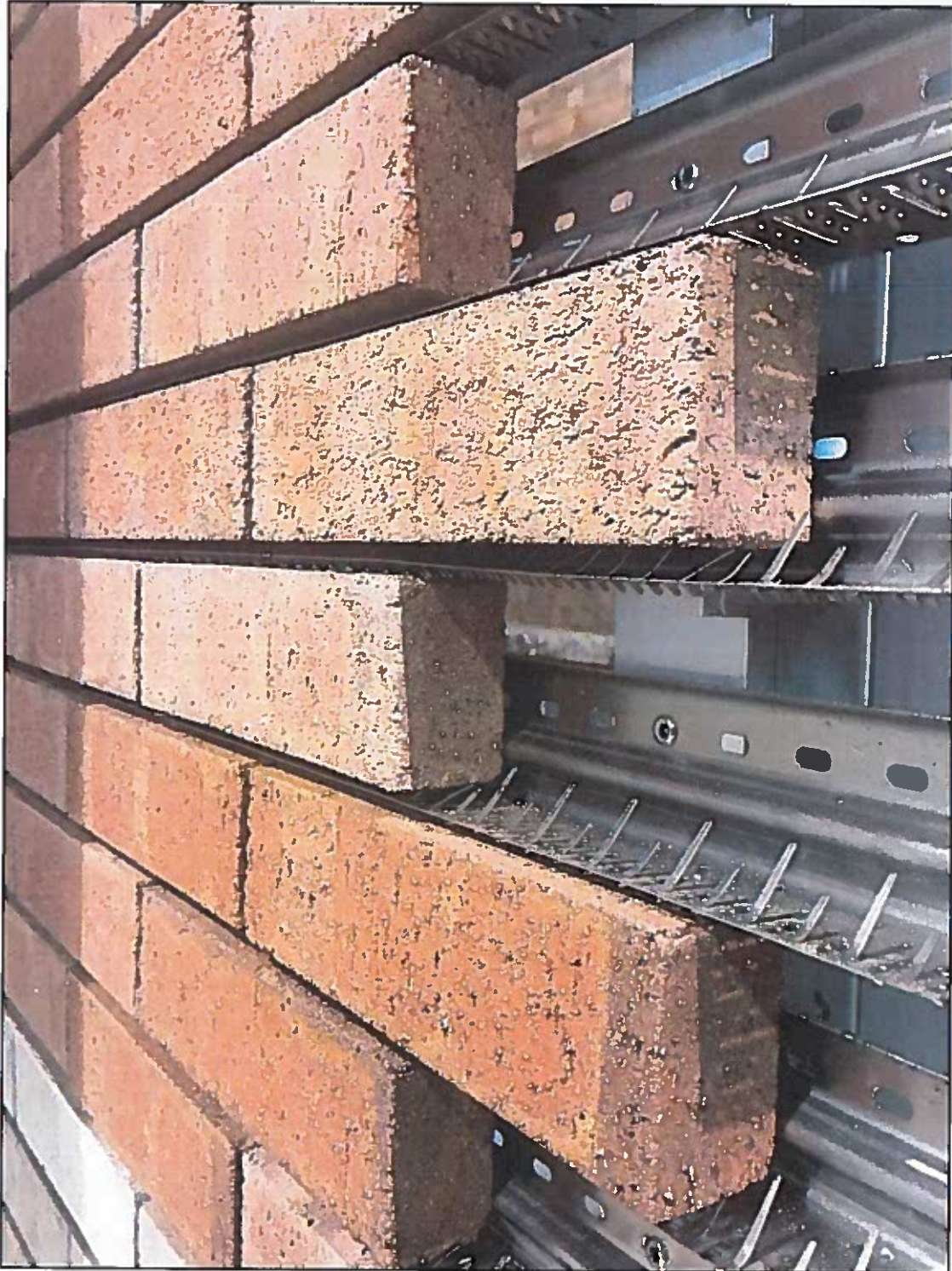
CLOSE UP OF BRICK SLIPS
