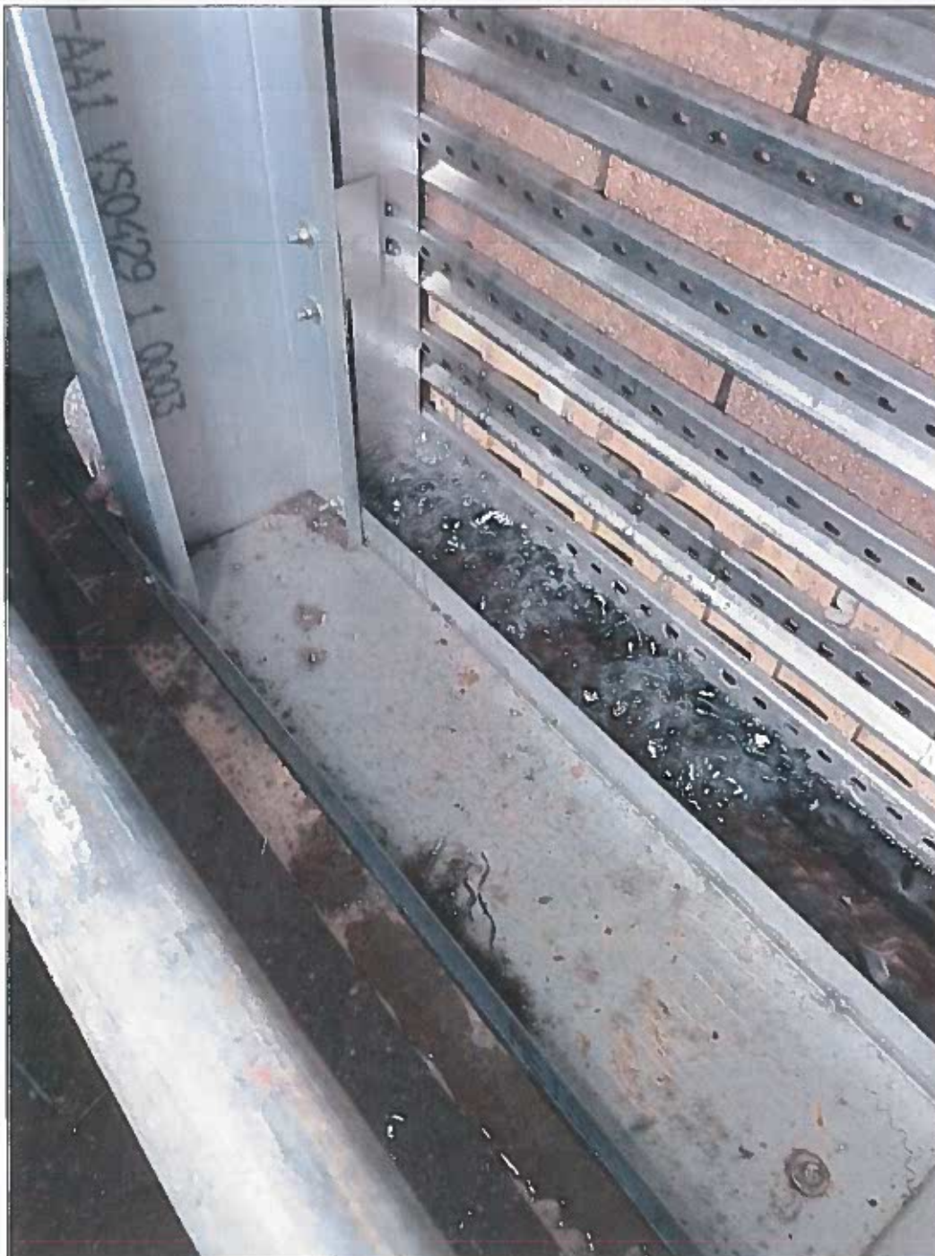
INTERNAL VIEW DURING WATER TEST
