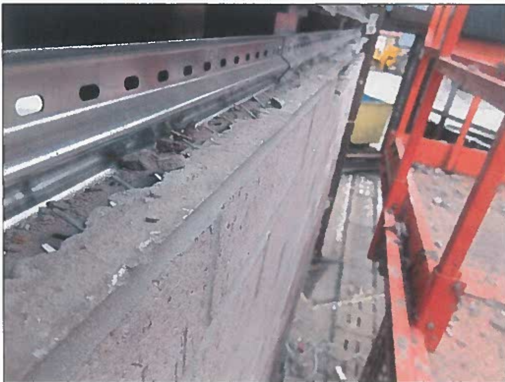
TEST SAMPLE DURING DISMANTLE
